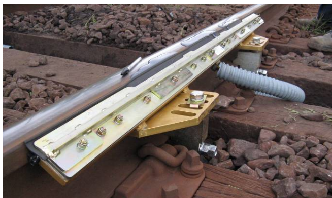
Figure 9 – KELTRACK friction modifier applied by TOR-XL on MRS Track
