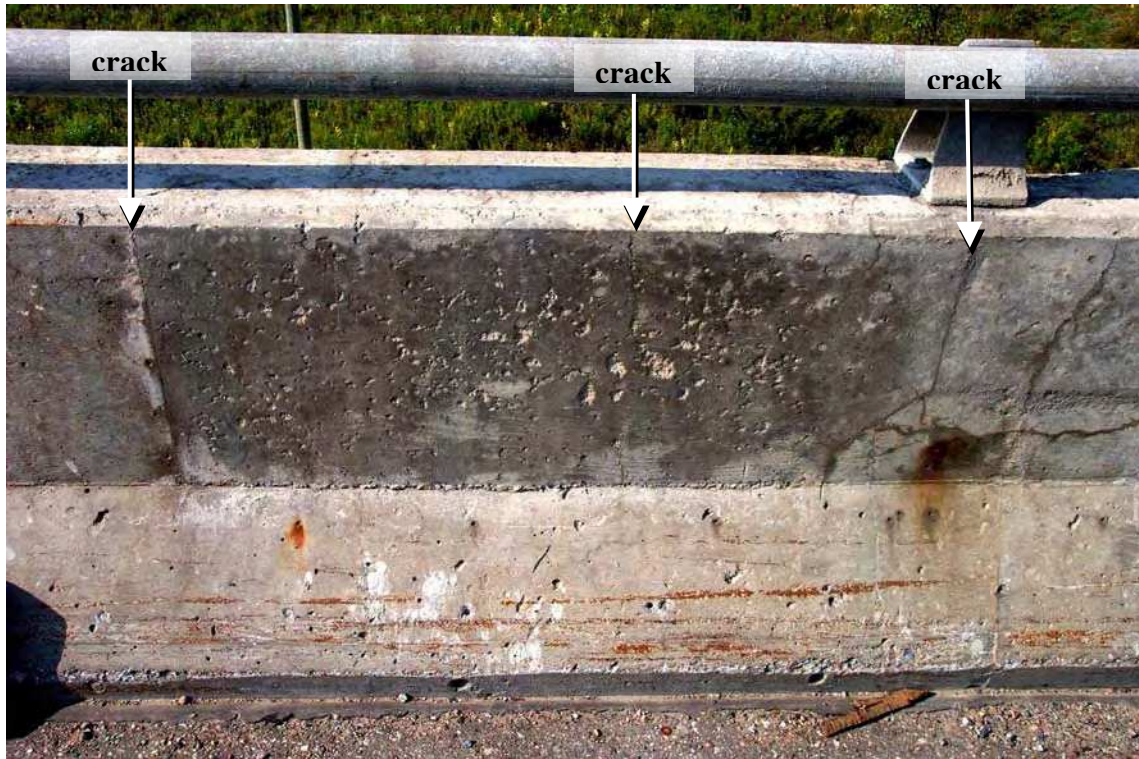
Fig. 13 – Photograph of repaired Section 2 after four years (Oct. 2003)
