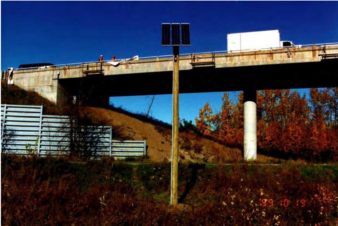
Fig. 1 – Test bridge during repair and instrumentation
