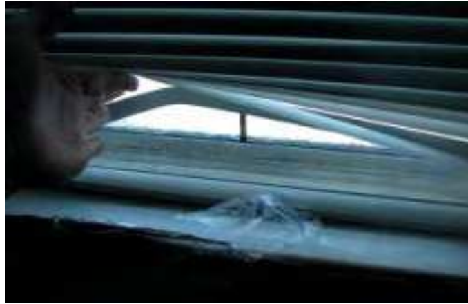
Figure 22 Excessive window condensation (Stad 2006)
