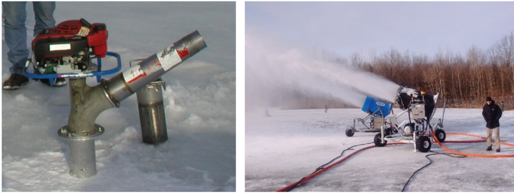
Figure 6. Ice cover thickening may be conducted using a pump to flood the ice (left) or implementing a spray ice system (right). Source: NRC.
