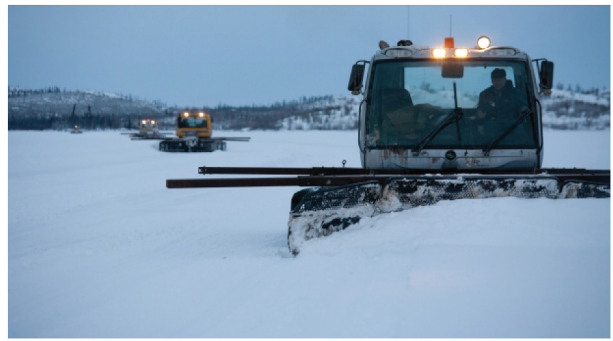
Figure 5. Snow cat plowing machines are preparing a winter road operation for opening. 6
