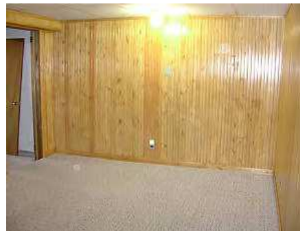
Figure 16. Combustible (wood) wall finish
