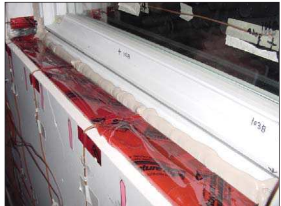
Figure 8. Sealing the window frame to the air barrier at the interior side
