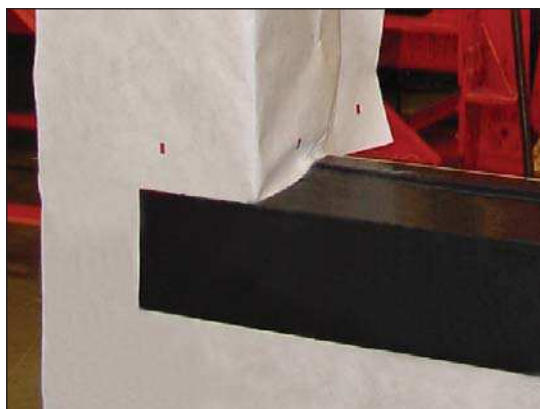
Figure 7. Proper lapping of sheathing membrane and self-adhered flashing (shingle fashion)
