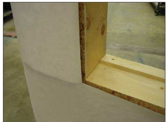
Figure 5. Sloped sill and back dam
