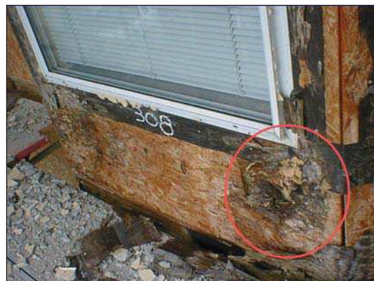
Figure 1. Damage caused by water entry
