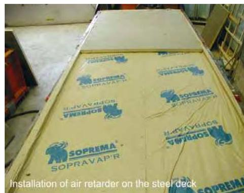
**Figure 9: Typical layout of assembly with air retarder**
