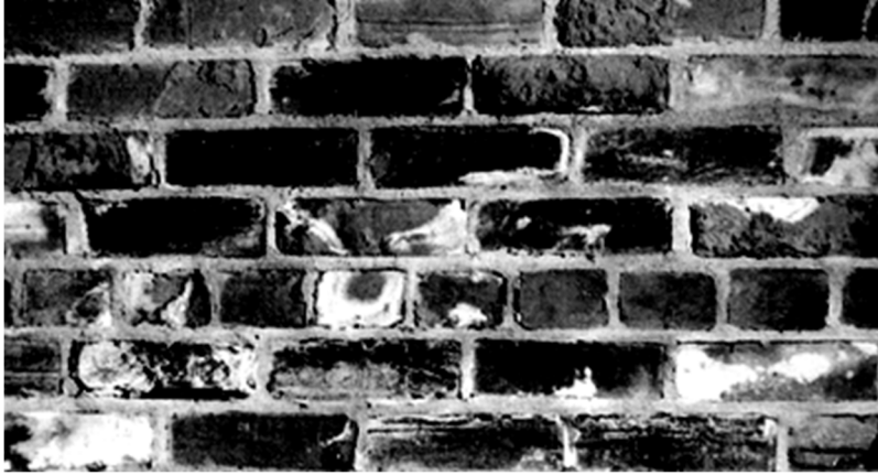
Figure 1. A wall built of bricks recovered from the demolition of old buildings damaged after one year of service by the spalling of many bricks and marked by efflorescence.
