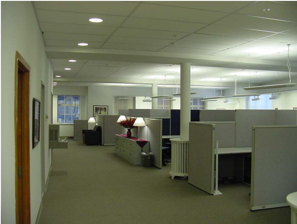
Figure 1. General view of cubicles with a single dimming direct / indirect luminaire centred over each cubicle and wall washing around the edge of the space.
