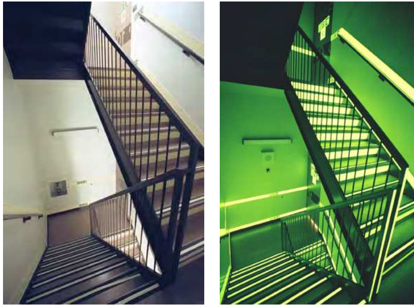
Figure 4: Stairway C with PLM marking, lights on and off, First Study
