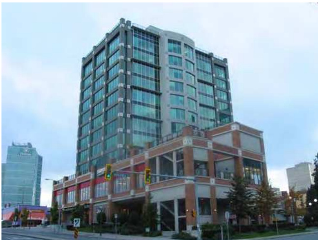
Fig. 1 North-east view of the test-site.
