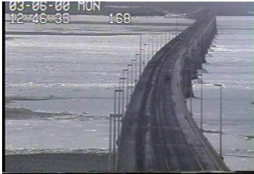
Figure 7 Ice piling on the bridge piers
