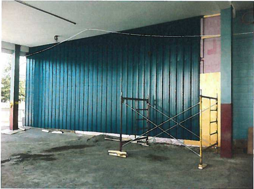
Figure 7. Insulation and siding.
