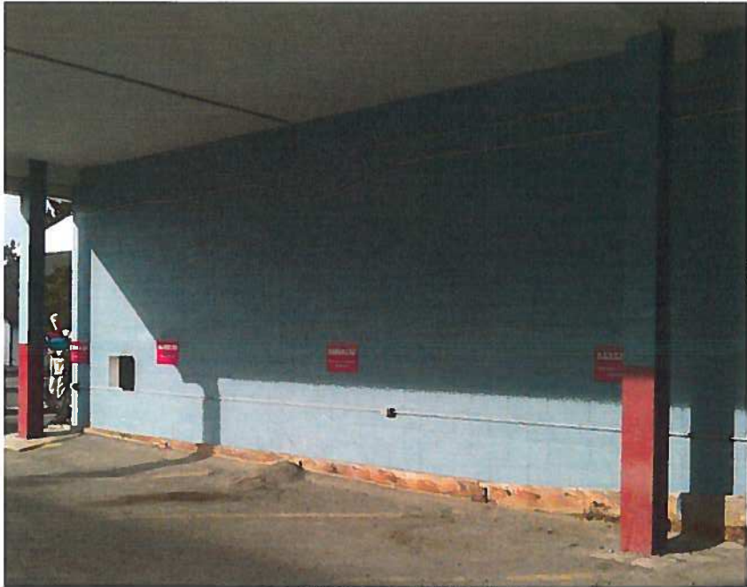
Figure 4. Wall selected for VIP retrofit project.
