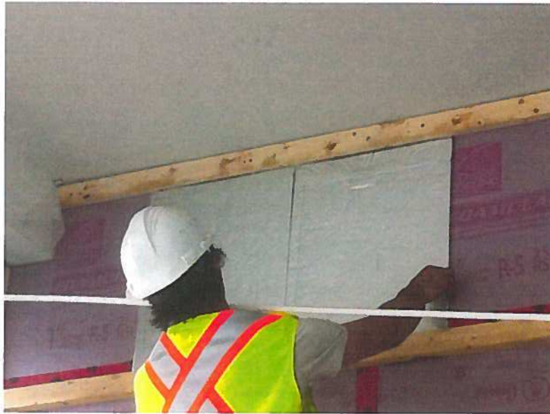
Figure 6. Installation of the vacuum insulation panels (VIPs).
