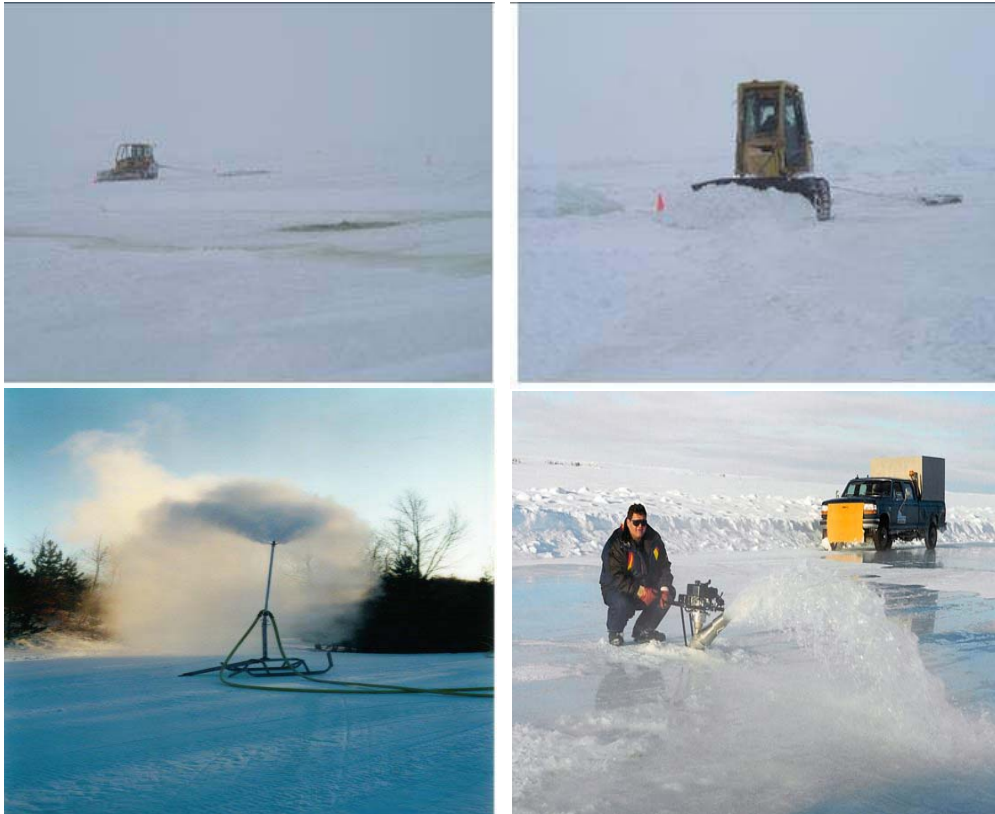
Fig. 5 D3 Cat, Snow making equipment and free-flooding pump.
