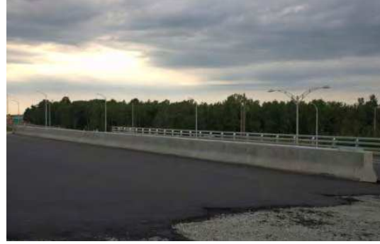
(b) After formwork removal
