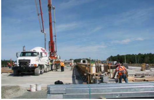
(a) During concrete casting
