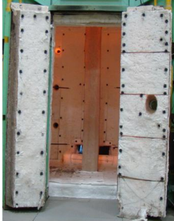
FIGURE 10. Column Specimen just after 4 Hours Fire Exposure.
