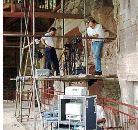
Figure 3: A 3D laser scanner on an unstable scaffolding structure; the working environment seriously compromises the accuracy of the range data.
