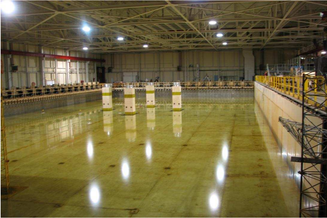
Photo 1: Column 1-2-3-4 are shown in the Offshore Engineering Basin (OEB) of NRC
