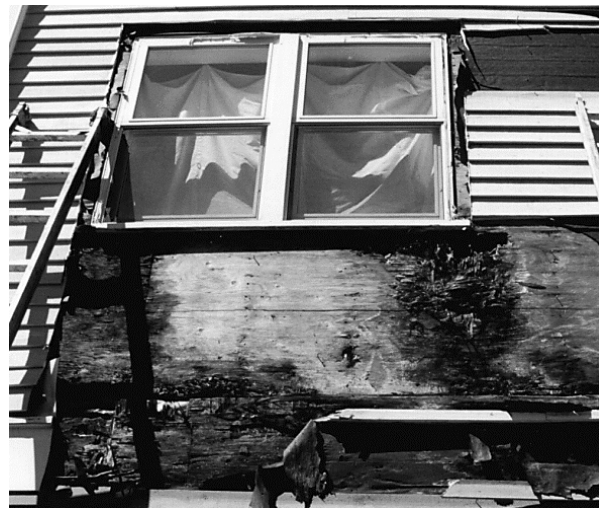
Figure 2. Pattern of damage to the sheathing board underneath the windows (Project B)
