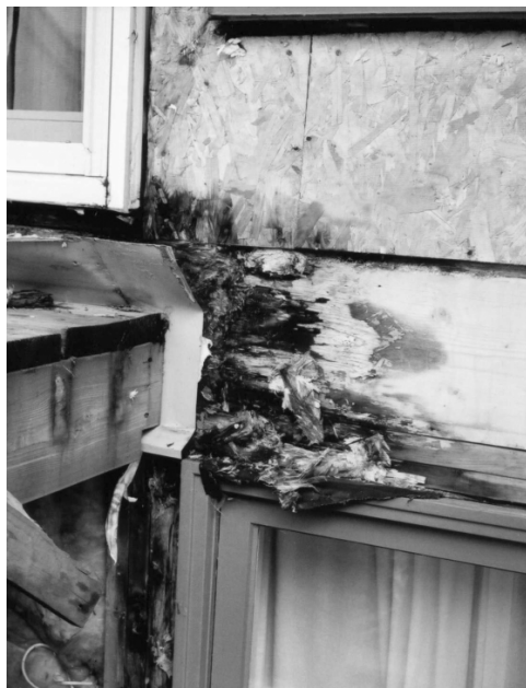
Figure 4. Flashing is in place, but is crushed between the wall and the ledger board, resulting in little potential for water drainage on its face (Project A)
