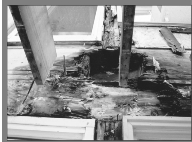
Figure 1. Damage to the wall elements adjacent to a balcony joist/wall connection
