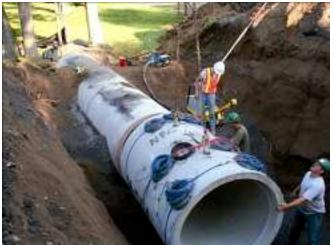
normal pressures at the maximum and minimum points in the Heger pressure distribution. In addition, four earth pressure cells were installed in the embedment soil at the top, springline and bottom to measure soil pressures that are perpendicular to normal pressures. The plane of the pressure cells corresponds to the plane of the embedded strain gauges for both test pipes.
