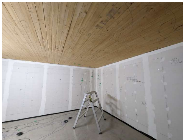
Figure 2: Walls and CLT ceiling in one of the lower rooms of the flanking facility
